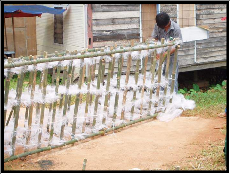
Fig. 5 Biomedia Frame under construction
