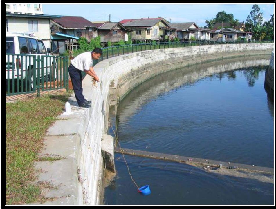
Fig. 7 Progress Photos Taken In December, 2006
