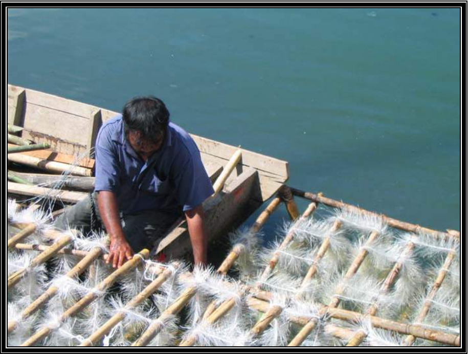
Fig. 6 Installation Of Biomedia
